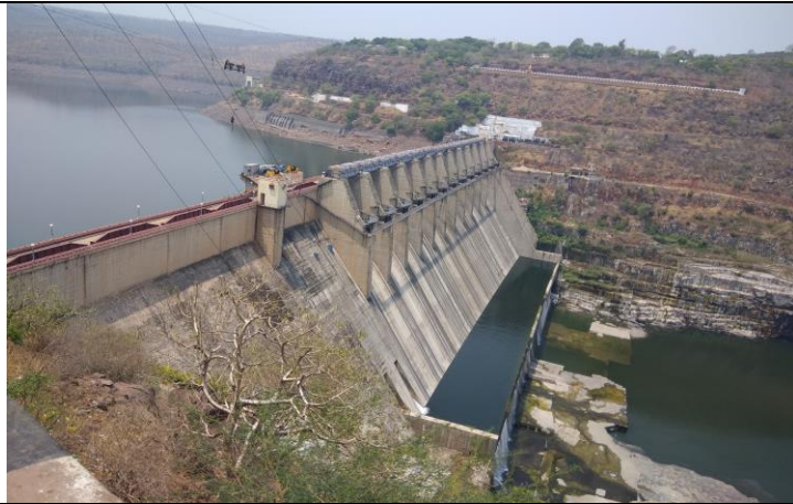
Srisailem Right Bank Power House
